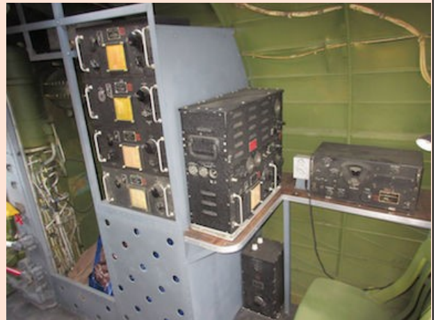
Radio Operator's Station
